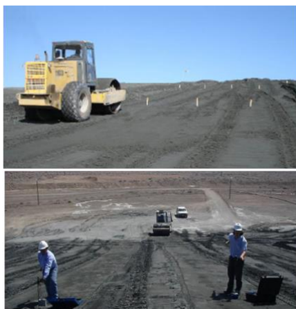
Figure 10a - Slope compaction control
