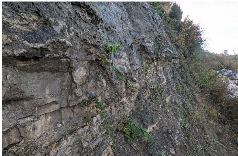
Section of visible rock beneath recent mantle failure
