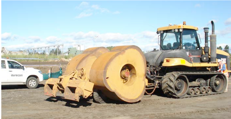
Photo 1: Landpac 17.5t 3-sided impact roller used in field compaction trials.
