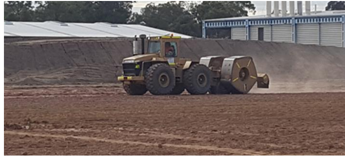
Figure 3: Tractor and pentagonal drum used
