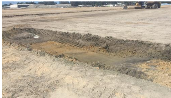
Figure 4: Removal and replace of areas post proof rolling
