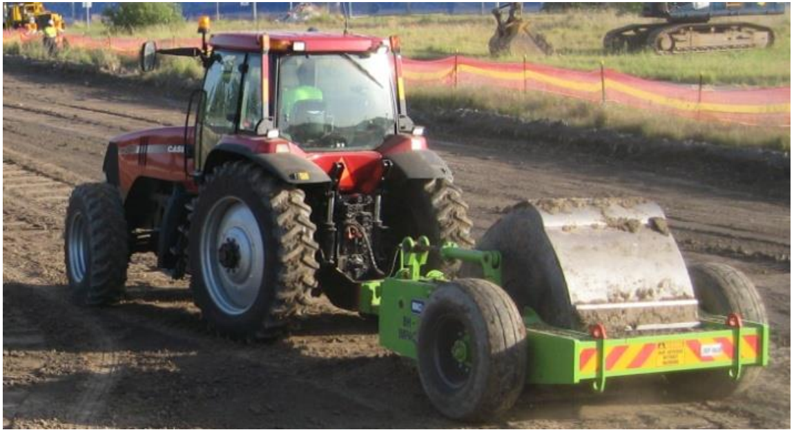
Figure 2. Impact rolling in progress.
