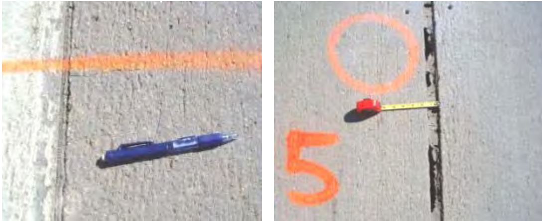
Figure 14. Control Joint A (left) with low-severity crack above a tie bar and Test Joint B (right) showing the sealant detached and with 1¼-in. opening.
