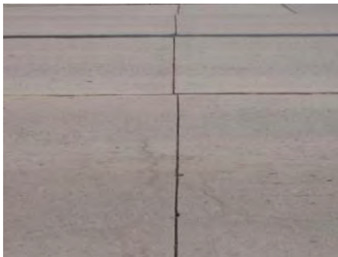
Figure 3. Slippage between lanes as evidenced by misaligned transverse joints in adjacent lanes.
