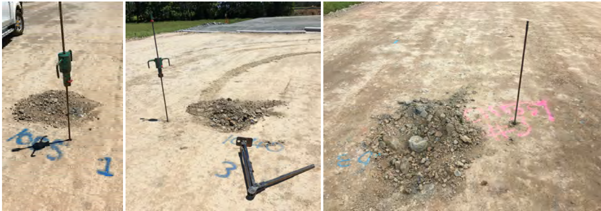
Figure 7-11 Pictures of the DCP equipment typically adopted onsite, with testing locations shown in close proximity to the sampling locations associated with the traditional QA assessment undertaken
