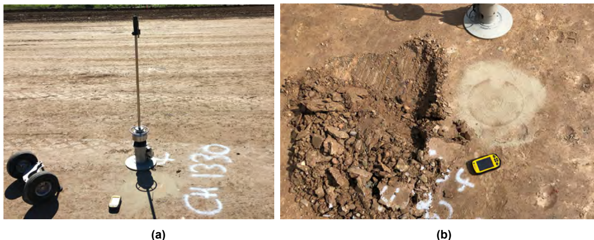
Figure 7-4 (a) Picture of the 'Prima 100' LWD equipment typically adopted onsite, fitted with 300 mm diameter plate; and (b) minimal bedding sand and circular indentation of plate typically observed at conclusion of 'Prima 100' testing (note also limited offset between LWD and material sampling site from side-by-side density and field moisture content assessments)
